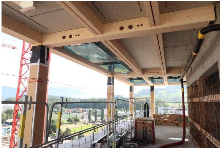
Figure 7.11 Examples of edge beams with holes for installations in the Arbo building.
