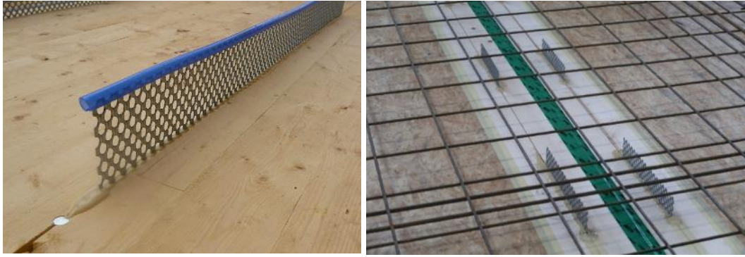
Figure 2.12 HBV glued in connector and casting process for a prefabricated timber concrete composite slab (Photos: Erne AG, TiComTec GmbH)
