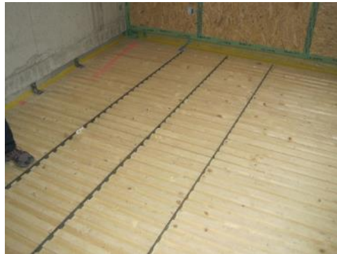
Figure 2.11 Examples of flat-steel-locks
