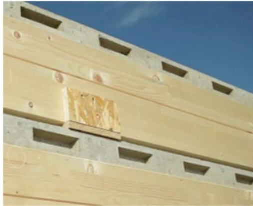
Figure 4.3 Recesses in the concrete (Image Copyright: CREE GmbH, www.creebuildings.com )
