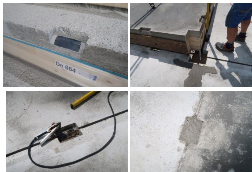
Figure 4.1 Welding of floor elements in the Suurstoffi S22 building
