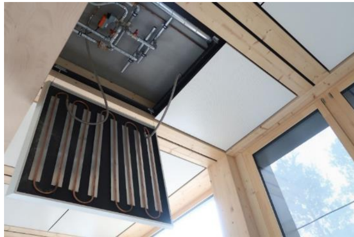
Figure 7.10 Examples of accessing the bays between the ribs of floor elements with various installations in the Arbo building and Suurstoffi S22.
