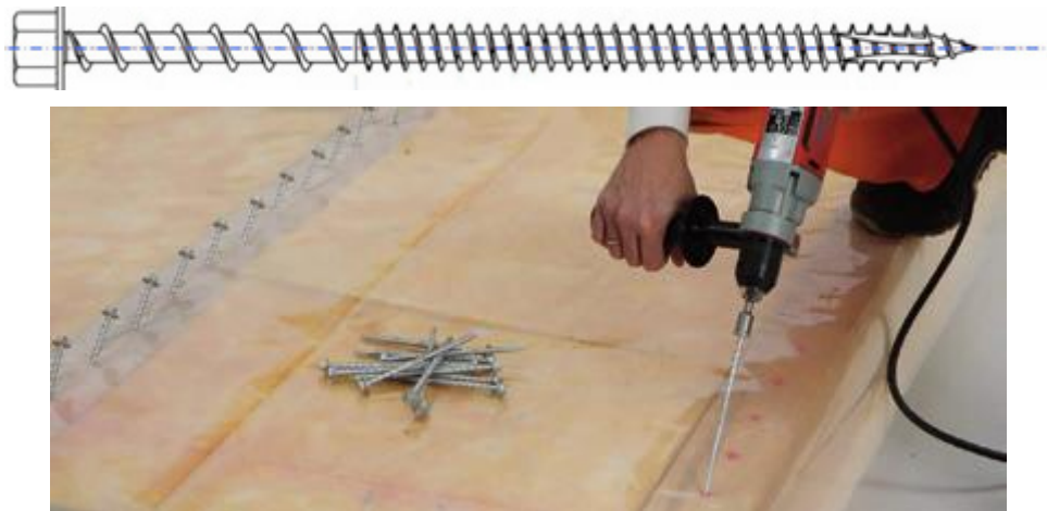
Figure 2.5 Drawing of SFix screw and photo of insitu application (Elascor 2021).
