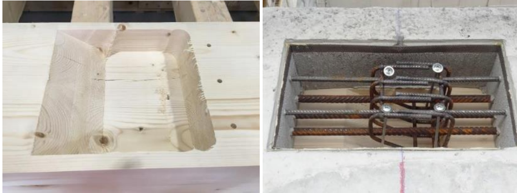
Figure 3.6 Notches in the timber and corresponding recess in the concrete slab over the ring beam spanning between the façade columns (Jung 2018).
