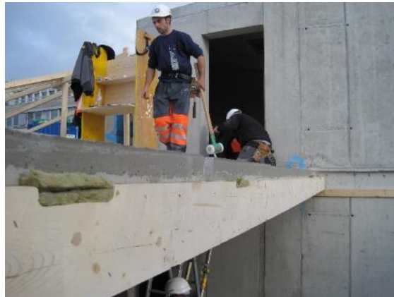
Figure 2.15 Prefabricated TCC elements with Brettstapel timber elements.
